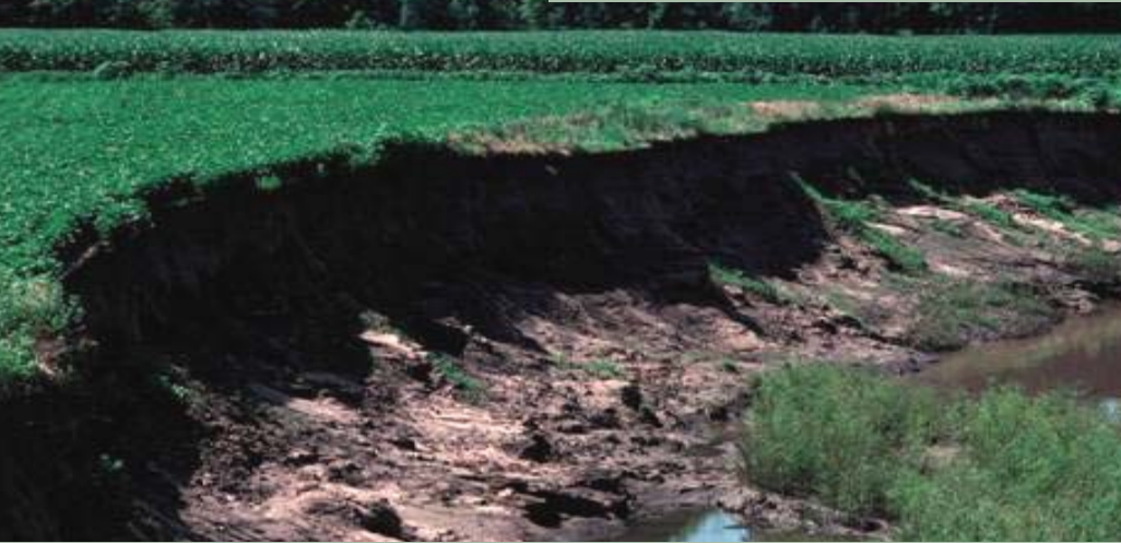
Bank Channel Erosion
