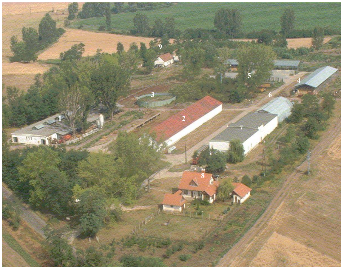
Figure 1: View of Józsefmajor Experimental and Demonstration Farm
