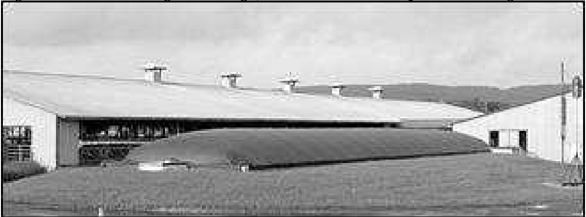
Figure 2.2: Anaerobic digestion design, membrane covered liquid manure lagoon
