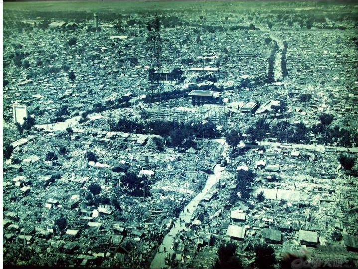
Figure 1: Tangshan shortly after the earthquake (China Earthquake Administration)
