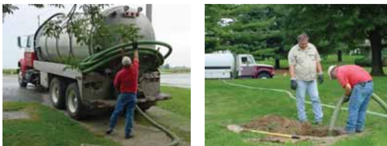
Figure 5. Emptying of the Septic Tank
