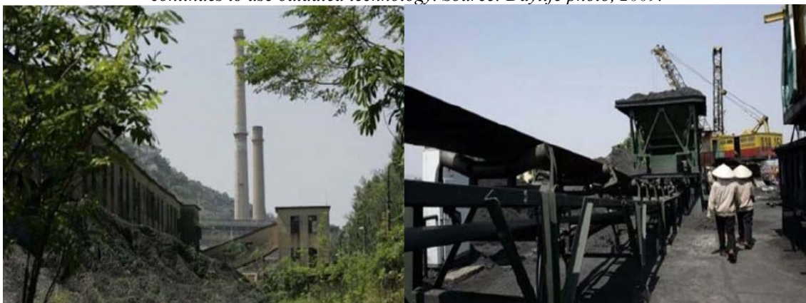
Figure 1: The Ninh Binh conventional coal-fired power plant was constructed over 20 years ago and continues to use outdated technology. Source: Daylife photo, 2009.
