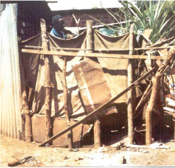
Unroofed flimsy latrines ("passport size")
