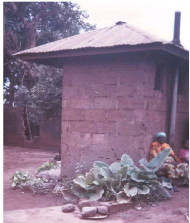
High standing latrines (VIP)
