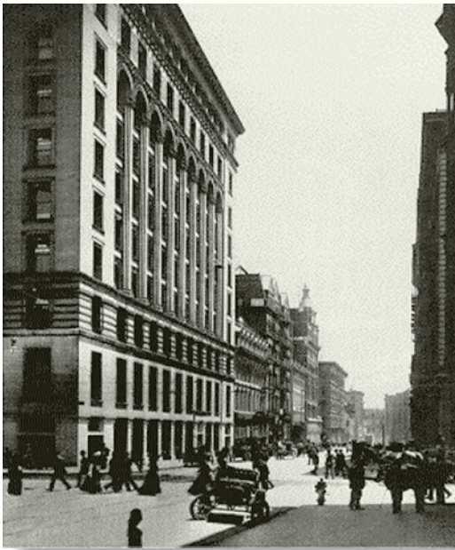
San Francisco's financial district, Bush Street Courtesy, California Historical Society, San Francisco
