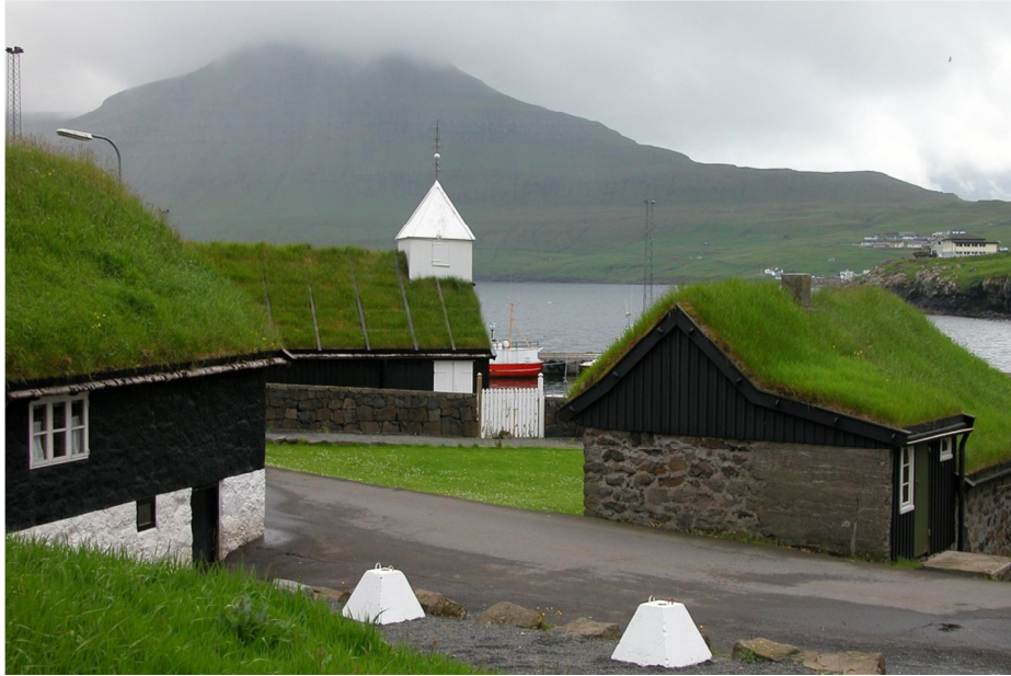
Picture 35: Traditional sod roofs – Scandinavian type of green roofs, which can be seen at numerous places in Faroe Islands. (source: Erik Christensen, https://en.wikipedia.org/wiki/Green_roof#/media/File:Nor%C3%B0rag%C3%B8ta,_Faroe_Islands_(2).JPG )
