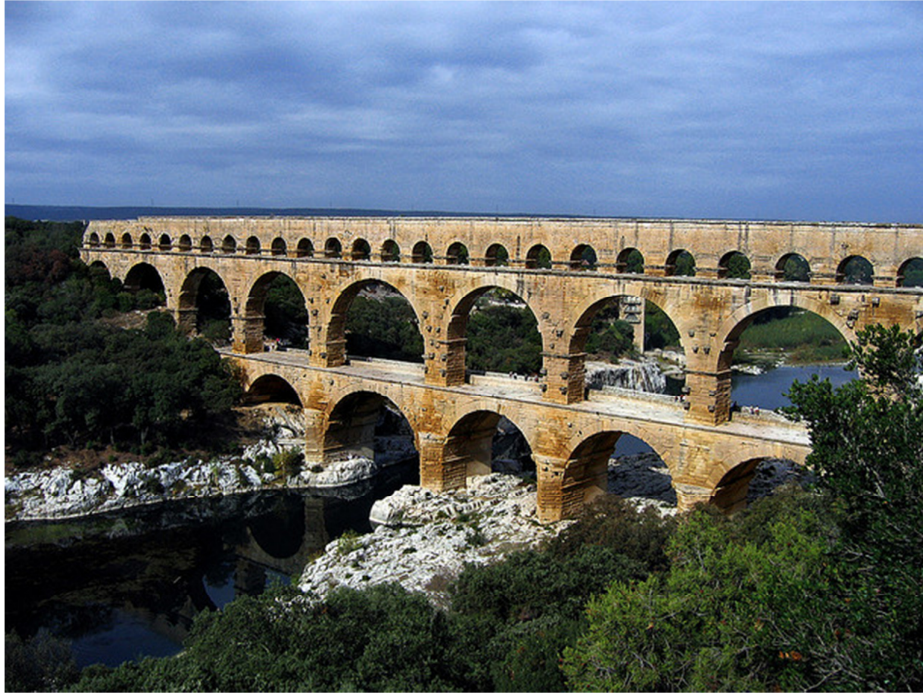
Picture 4: The Pont du Gard is an ancient aqueduct in the South of France built by the Roman Empire. It was initially part of a 50 kilometres long canal, supplying fresh water to the Roman city of Nimes. (source: http://www.touropia.com/ancient-aqueducts/ )
