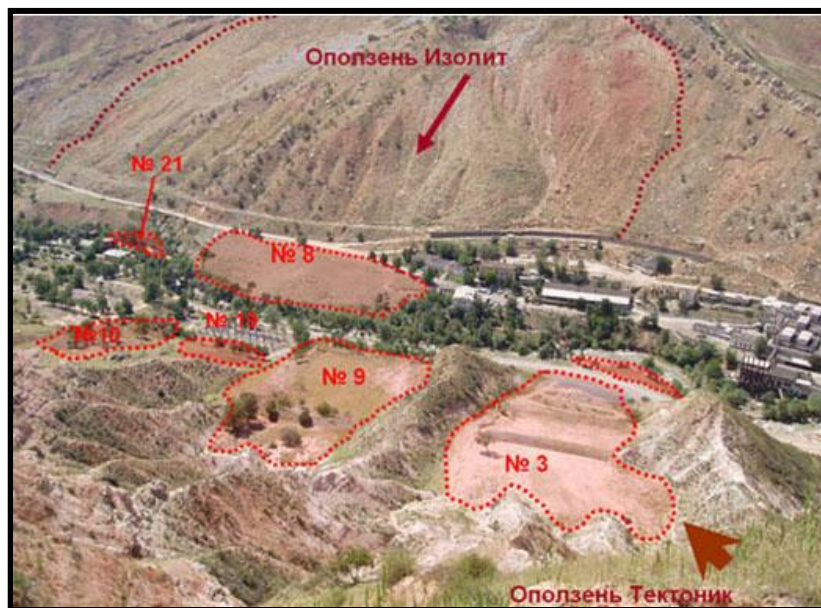
Fig. 7 Tailing Dumps at Maili-say 13
