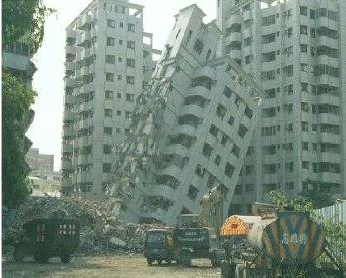
Figure 8: The Fall of the Twin Margalla Towers in Islamabad
