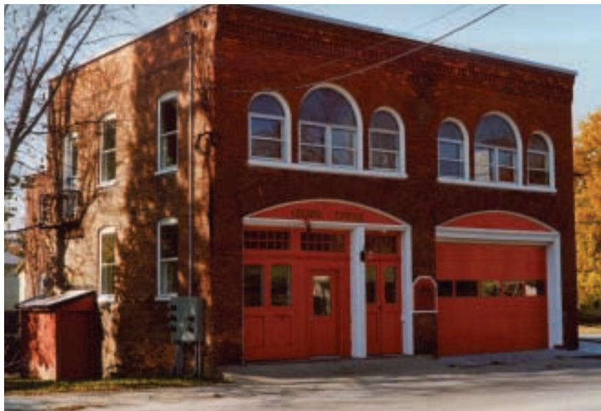
Putting adaptive reuse to work, the Vermont Arts Exchange restored two nineteenth-century firehouses in Bennington with funding that included VHCB grants. The bottom floors were converted into gallery space and the top floors into housing.
