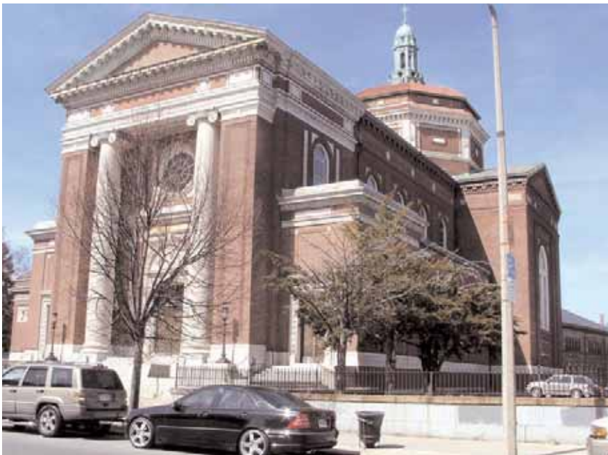
The Jamaica Plain Neighborhood Development Corporation purchased the Blessed Sacrament Church from the Archdiocese of Boston in September 2005. The renovation will provide for affordable housing, commercial space, and other community uses.
