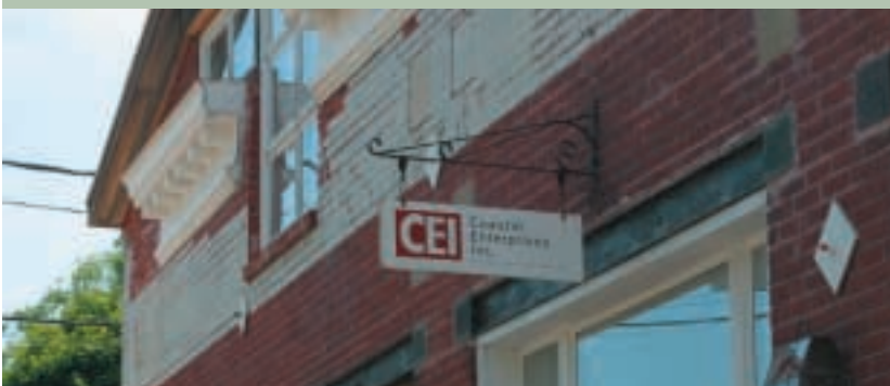
A former motor garage in Wiscasset, Maine, is the base of operations for CEI.
