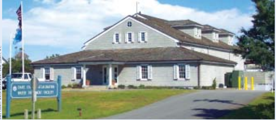
Parts of coastal North Carolina depend on desalted groundwater to supplement their water supply. Dare County, N.C., has built three desalination plants over the last 14 years to support their burgeoning residential development and tourist trade.
