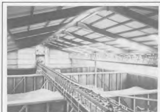
A typical aerated bulk store for paddy in Australia. Many countries of South East Asia plan to move from bag to bulk storage. ACIAR Project 8308 will tap Australian expertise in the in-store drying of bulk grain.
