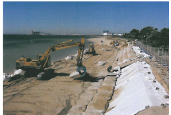
Figure 2 - Backstop wall under construction in Australia
