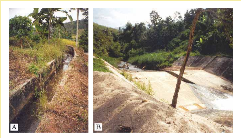
Figure 2.11 Examples of irrigation structures in sub-catchments of the Mae Chaem, northern Thailand: (A) a small irrigation canal in the Mae Pan sub-catchment; (B) a weir in the Mae Pan sub-catchment. Photos by W.S. Merritt, November 2000
