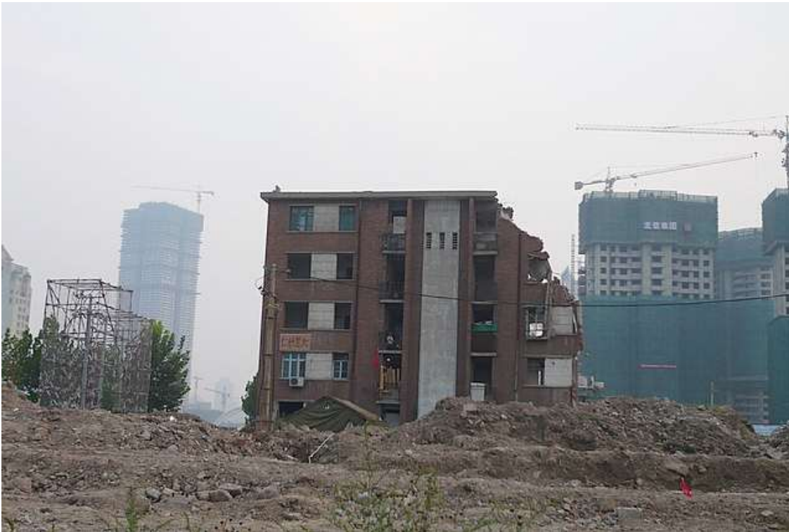
Figure 1: Defiant building standing alone in a cleared site of Tianjin © Hyun Bang Shin 2009
