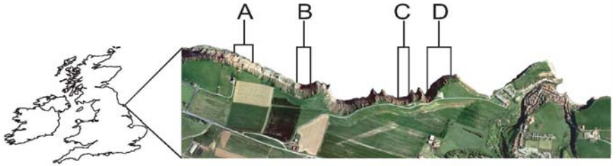
FIG 1. Location of monitored sites, Staithes, North Yorkshire.
