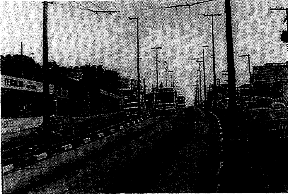
The São Mateus-Jabaquara has an extension of 33km of which 30 km are totally segregated busway
