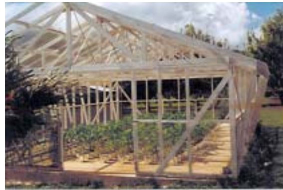
Figure 2.2 An open-sided greenhouse built for pot experiments in Tonga, which has a subtropical climate. Note the clear polycarbonate sheeting on the roof.
