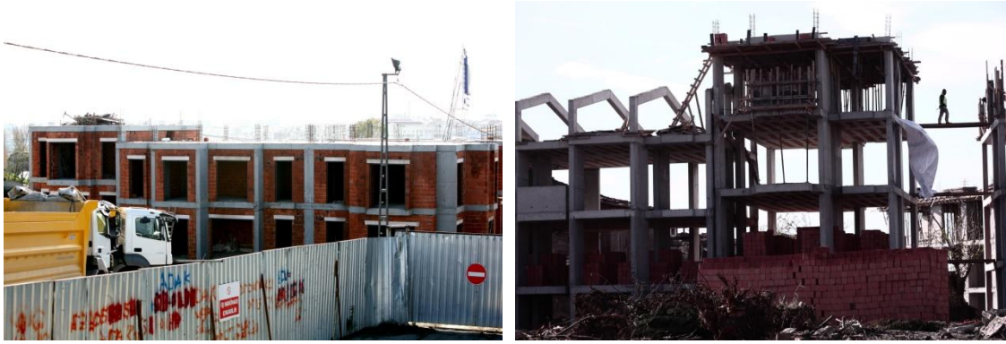
Photograph 2, 3: Construction of new and quotidian houses in Sulukule Photograph: Can Berkol, 25.11.2010
