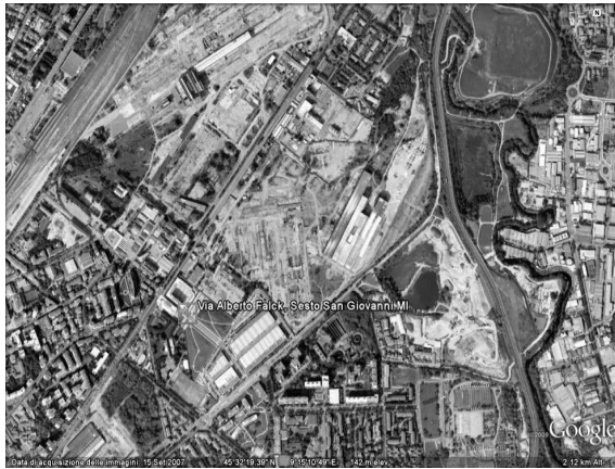
Fig. 1. Sesto San Giovanni. The brownfield of a huge steel industry in North Milan (Falck area).
