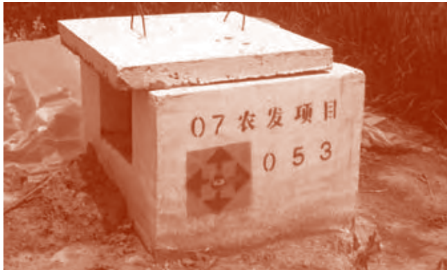
A covered well constructed from CAD program funds.
