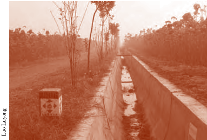
A cement canal constructed with CAD program funds.
