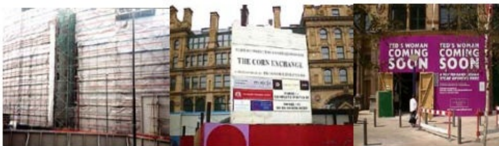
Images 3, 4 and 5. The Corn Exchange Building during the rebuilding process circa 1997- 2000
