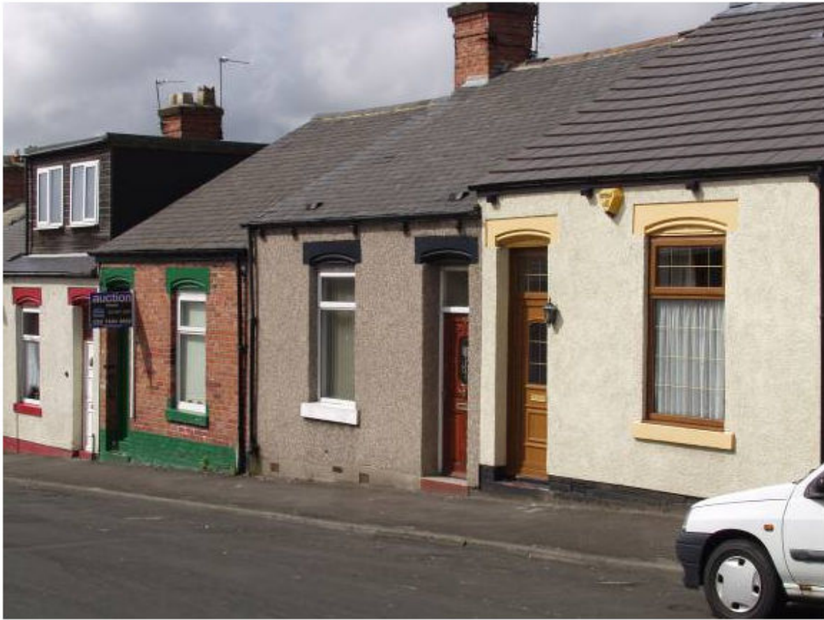
4.10 Because the basic house is so small the scope for enlargement, even when a dormer is built as in the bottom house here, is very restricted.
