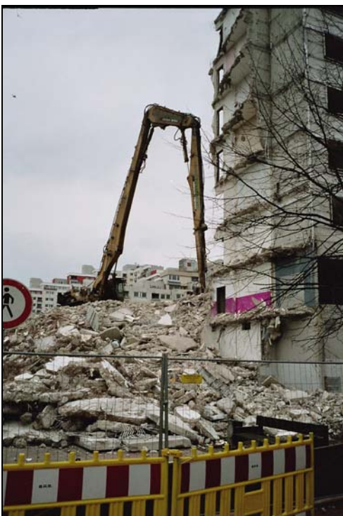
Fig. 21: Demolition of housing in peripheral estate of Osterholz-Tenever
