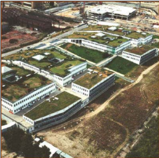
Figure 13: The Environment Park under construction
