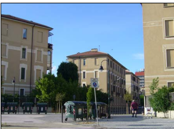
Figure 26: Upgraded housing, new pedestrianised area and new greenery in the previously dilapidated Via Arquata neighbourhood
