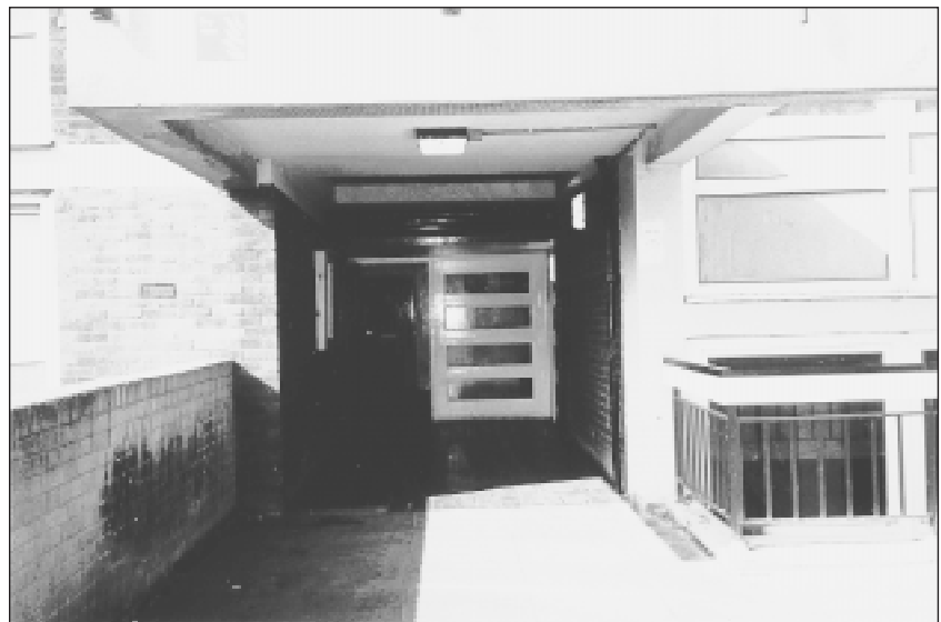
Insecure entrance to tower block
