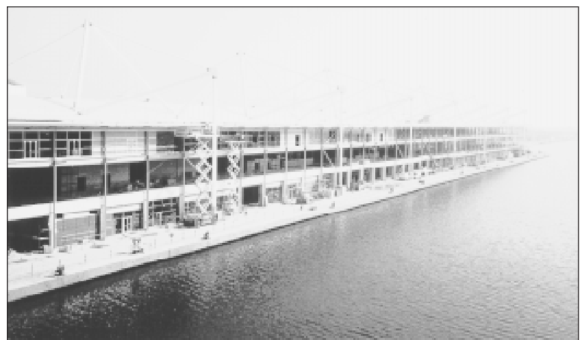
Construction of the exhibition centre
