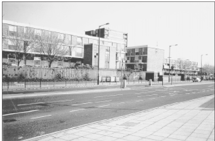
The fence along one side of East-Docks
