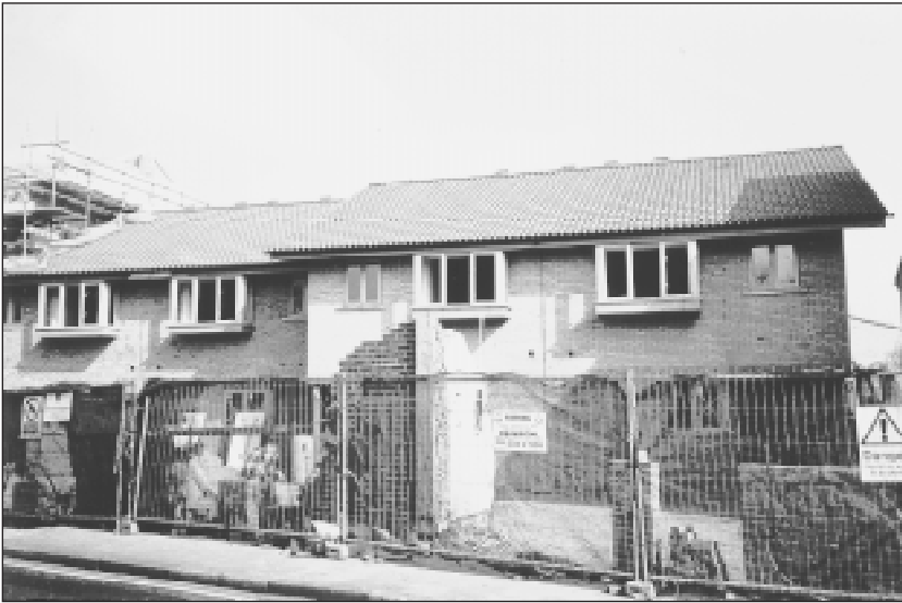
Houses being built for housing association shared ownership
