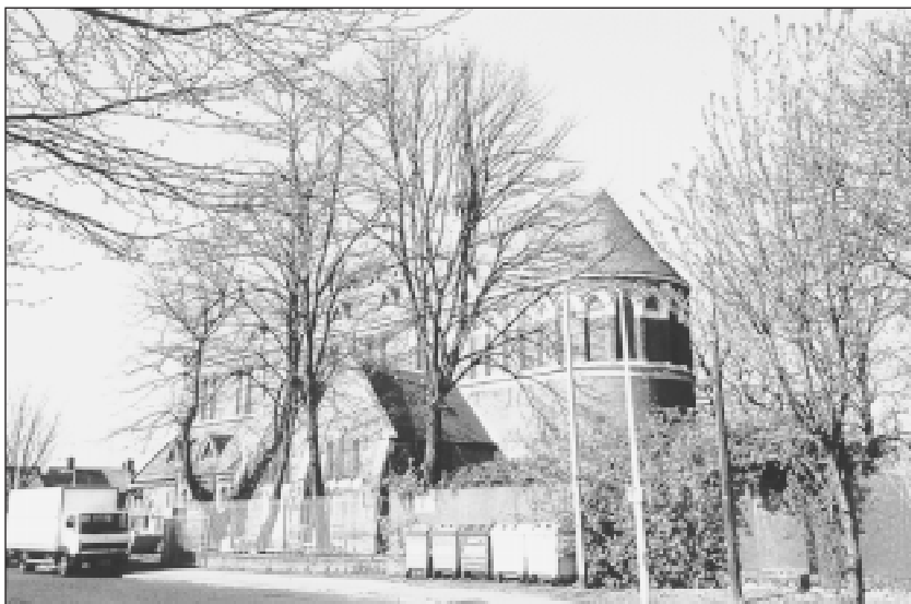
This converted church houses a whole range of community-led initiatives
