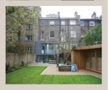
Traditional box sash windows had to be recreated to match the degraded original windows. They were then fitted with double-glazed sealed units and double draught seals were incorporated into the design to maximise energy efficiency.
