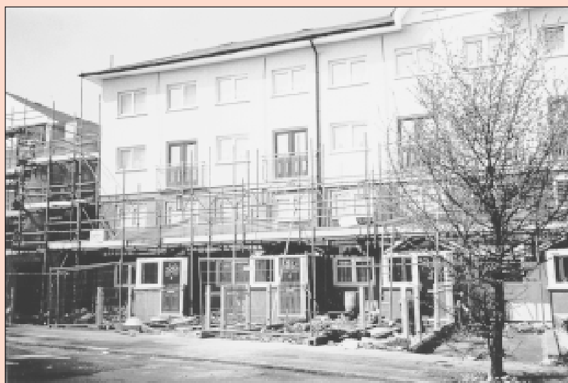
SRB-funded improvements in low-rise flats/maisonettes
