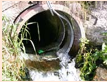
Figure 2. Subsurface hydrologic features in Sny Magill and South Fork watersheds. In the Sny Magill watershed (left photo), springs and caves discharge natural drainage from unknown areas of karst terrain. In the South Fork watershed, once-prevalent wetlands were converted to cropland with tile drainage. This 36-inch clay pipe (right photo) has discharged drainage collected from about 4,500 acres of cropland for nearly 100 years (note monitoring lines).
