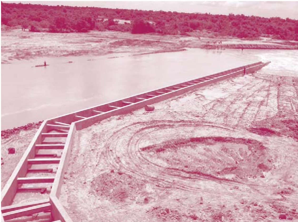
Figure 17: The fish pass of Stung Chinit reservoir (Photo E. Baran)
