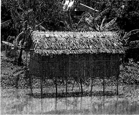
Poultry shed built with local materials (bamboo and nipa) for integrated poultry-fish farming.
