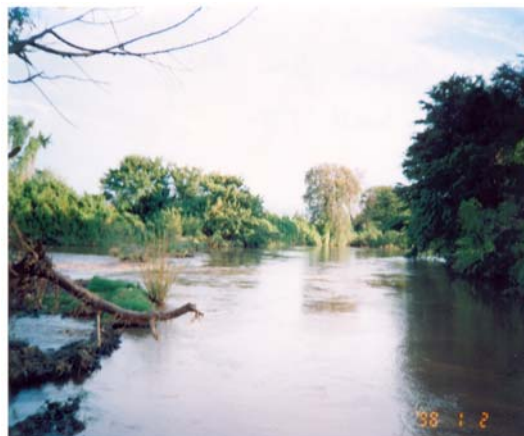
Diversion Weir at Nuraera
