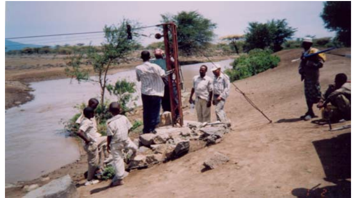
Preparation for work at Nuraera
