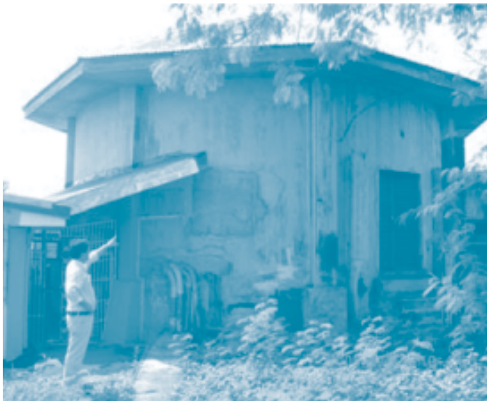
A concrete water reservoir of a water district in the Philippines.
