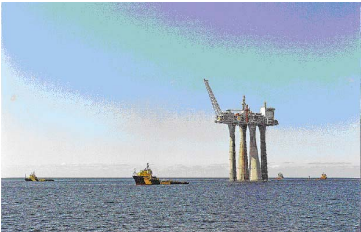
Figure 4: The largest Condeep ever built. The tow of the Troll A platform 1999 (Source: the Norwegian Oil museum)
