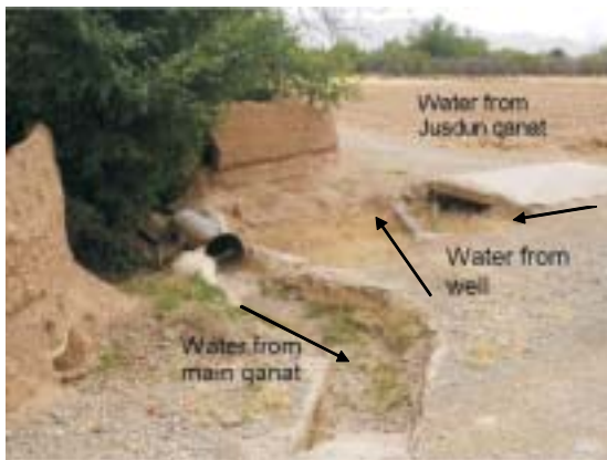
Example of intricacy in the distribution network
