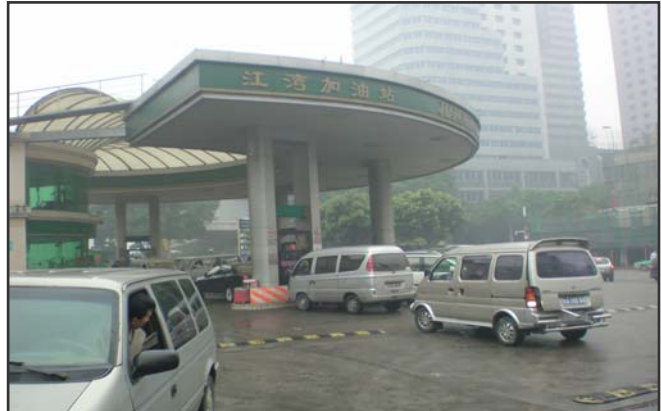
Fig. 4-4 Large Self-Service SS in Guangzhou
