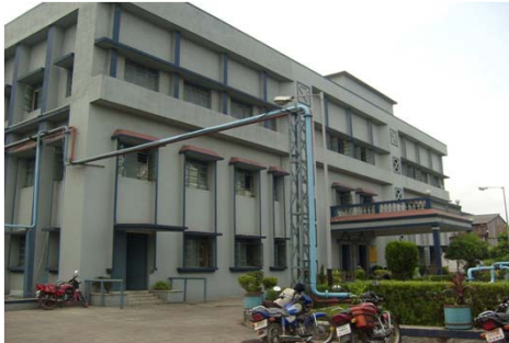
Front entrance to the main building
