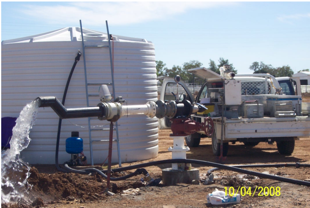
Photograph 3 Capping bore in Northern NSW
