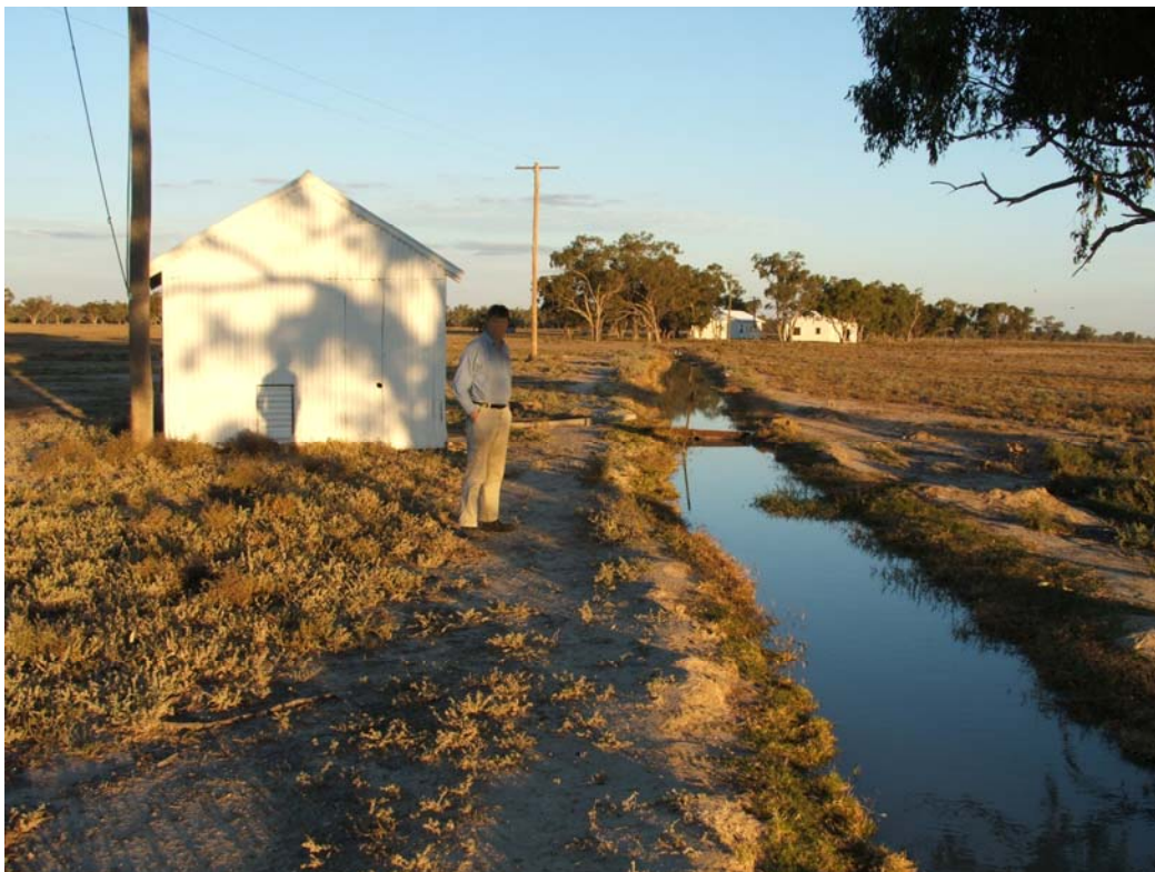
Photograph 4 Open Bore Drain Northern NSW
