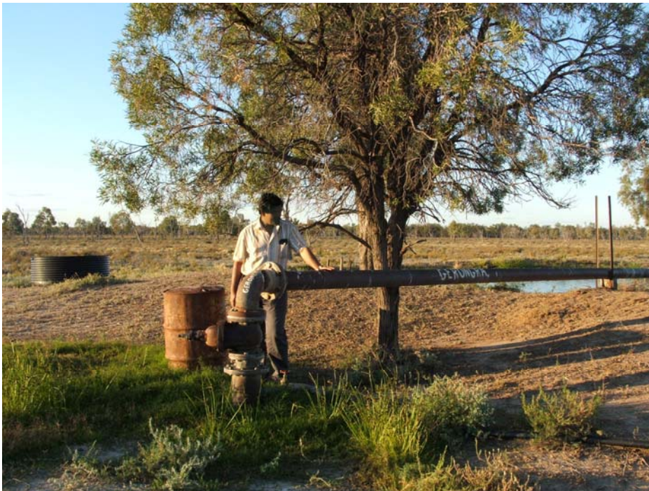
Photograph 2 Uncapped bore in Northern NSW with water flowing into drains
