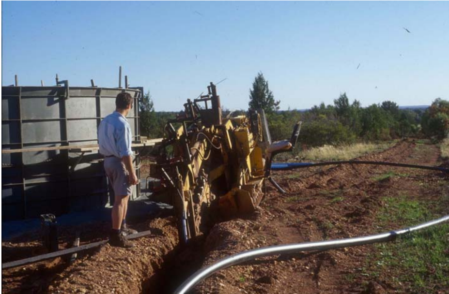
Photograph 1 Trenching for Piping in Northern NSW
