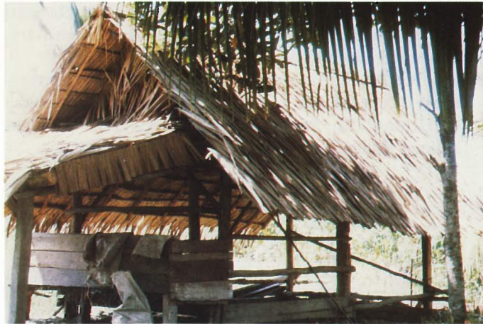
Photograph 1.5.2 An open-sided cattle house with a roof constructed with alang alang in Karang Agung Ulu, South Sumatera.
