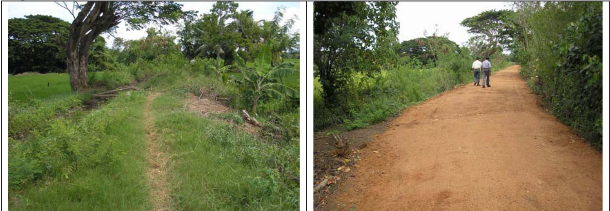
Figure 03: Access road to Paibokka anicut before and after rehabilitation
