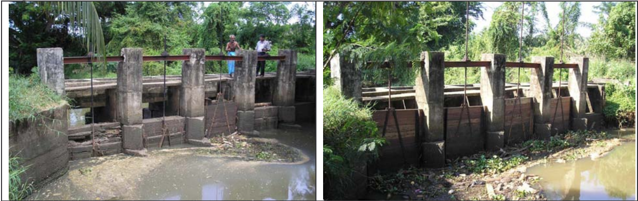
Figure 02 : Paibokka anicut before and after rehabilitation
