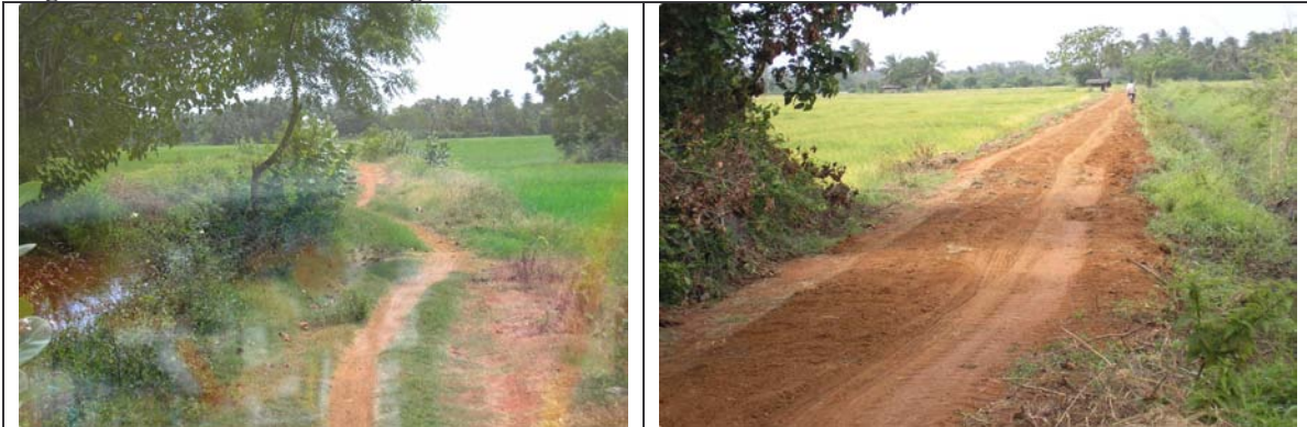
Figure 04: Access road to Karagas ara anicut before and after rehabilitation
