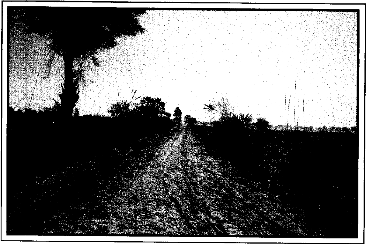
Photograph L. Inspection path from RD 27 to 31 after rehabilitation.
