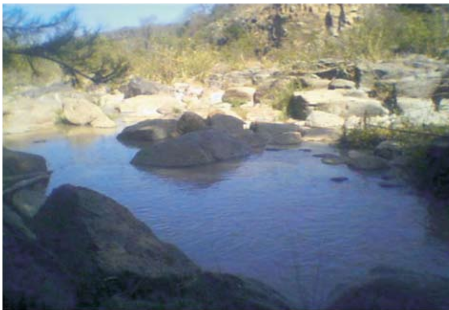
FIGURE 3. (a) Reservoir shoreline upstream of the dam; and (b) Seepage pools immediately downstream of the dam ( Photo credits: Jonathan Lautze ).
