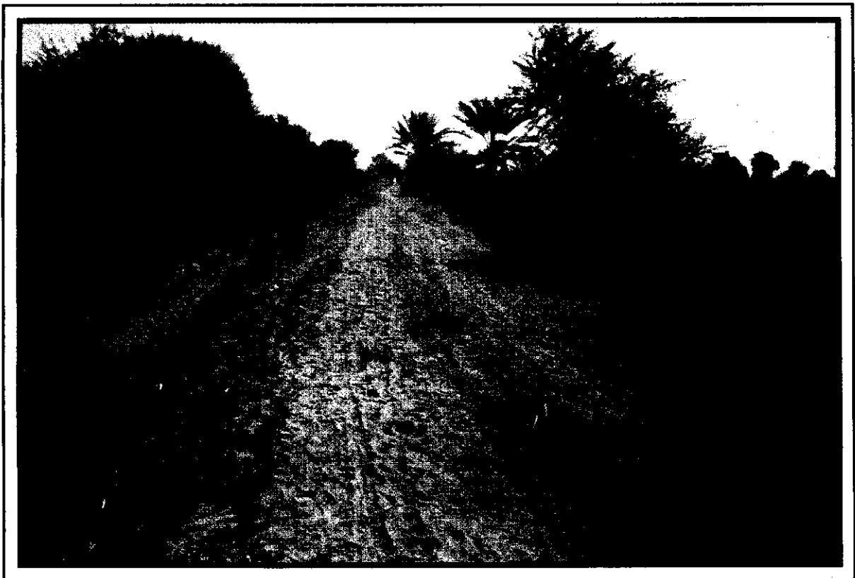
Photograph F. Rehabilitated inspection path.
