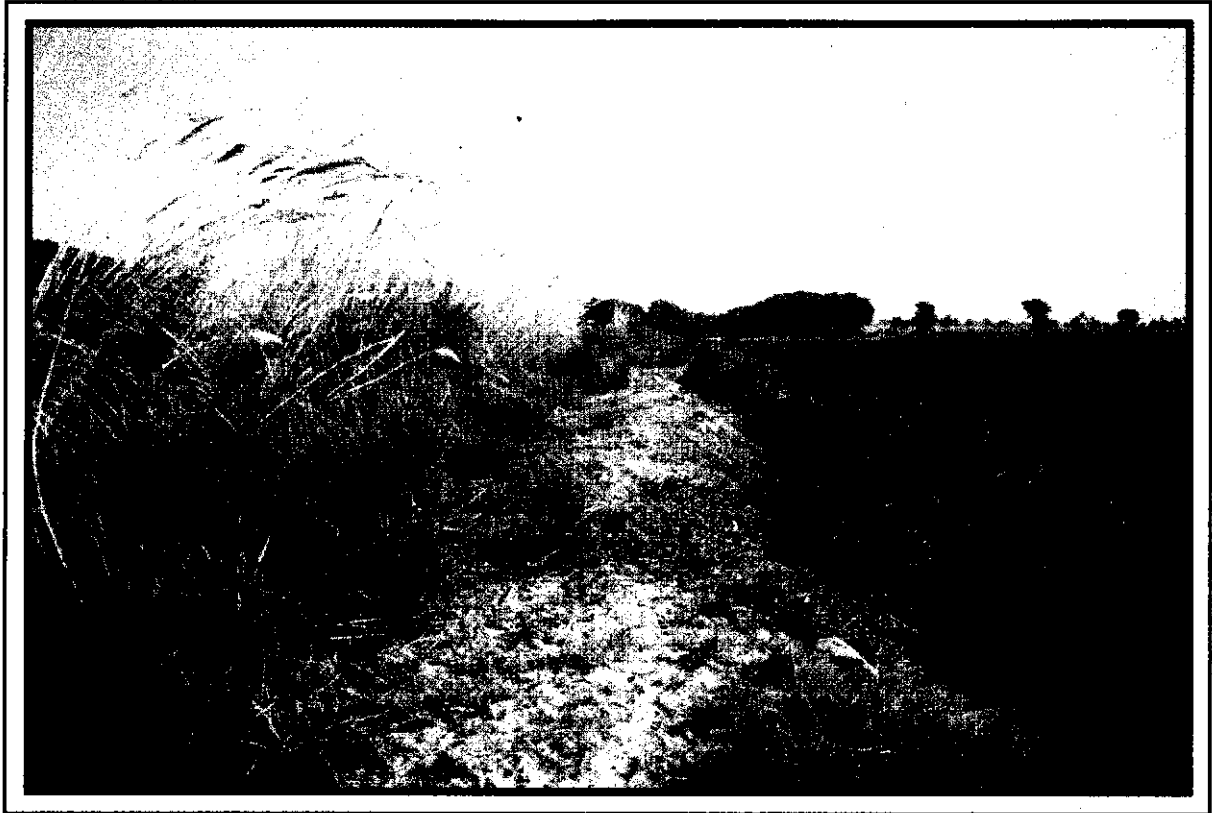
Photograph A. Condition of the channel before rehabilitation.
