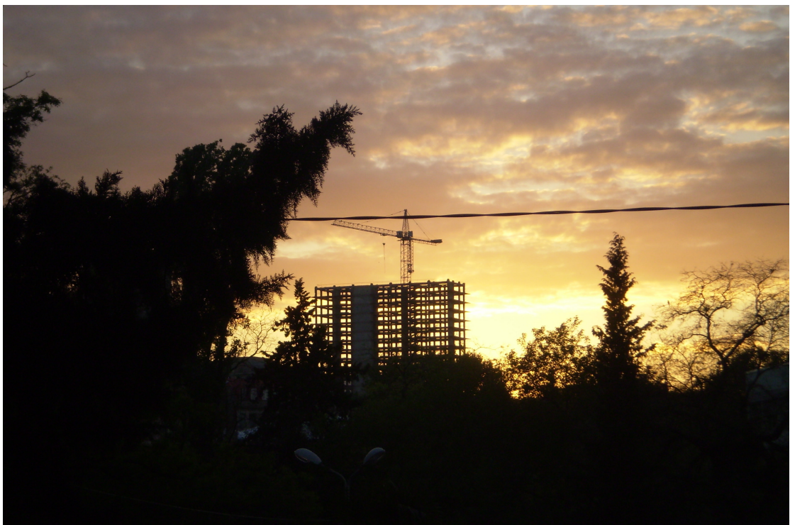
Photo 6: complete renovation of the former IDP-hotel Iveria
