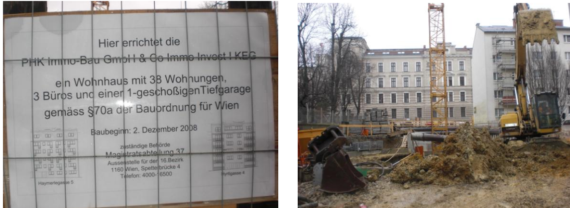
Figure 22. Ground-breaking Construction at Haymerlegasse 5 and Hyrtlgasse 4 in the Third Statistical District.
