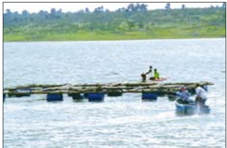
Figure 8. Installing frame at site
